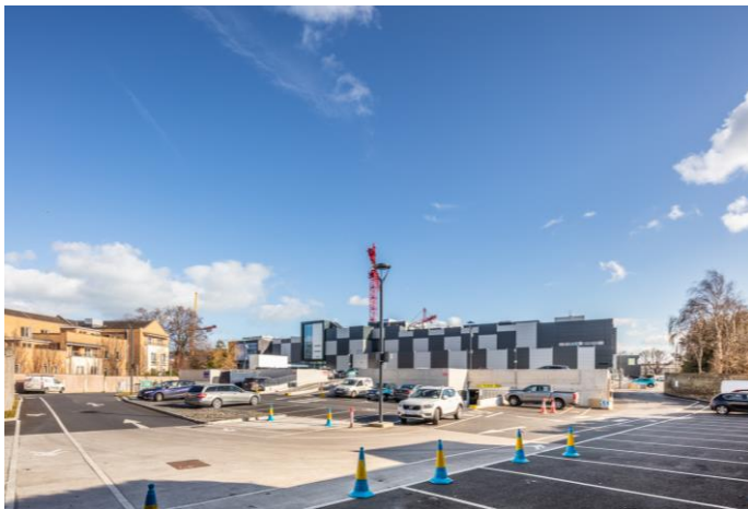
Existing view of car park deck from west
