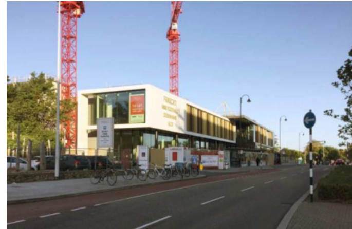
Existing view from east on Frascati Road
