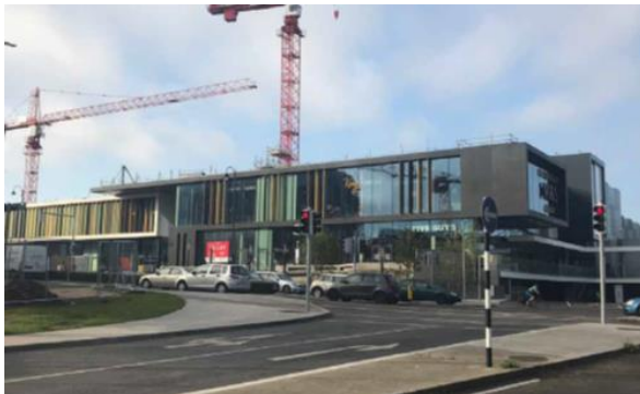
Existing view from north on Frascati Road
