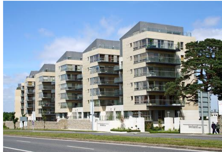
Example of existing apartment development by RA+U on the N11
