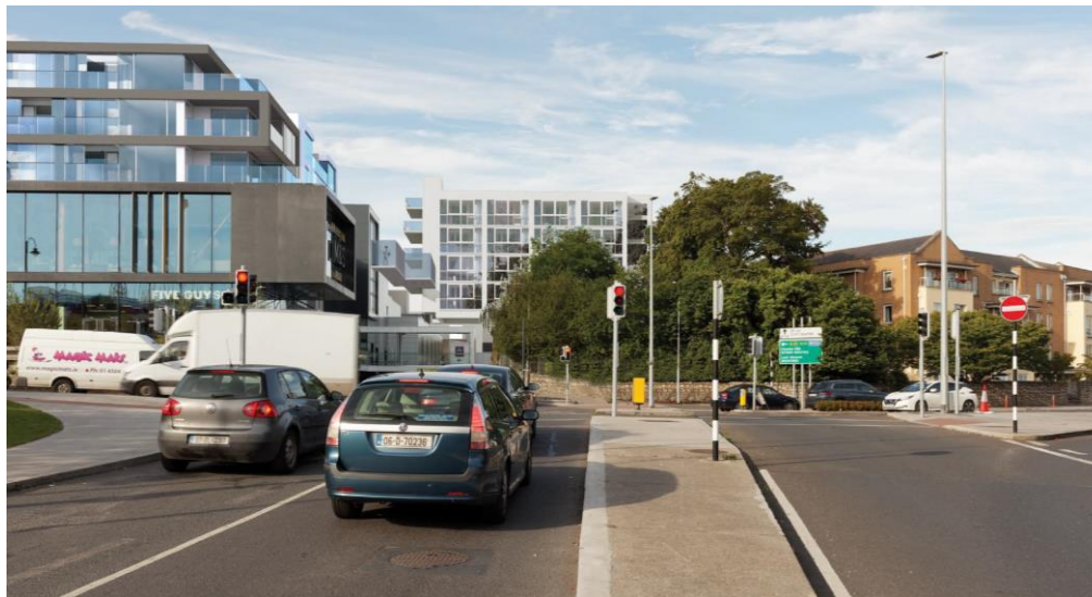
View of north east façade with permitted apartments facing onto Frascati Road and proposed additional phase 2 apartments set back over the existing car park decks
