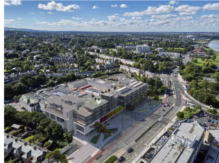
Aerial view from east of phase 1 apartments facing Frascati Road (prior to addition of additional apartments over car park deck for phase 2)
