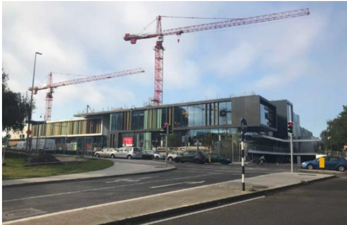
Existing view from north on Frascati Road
